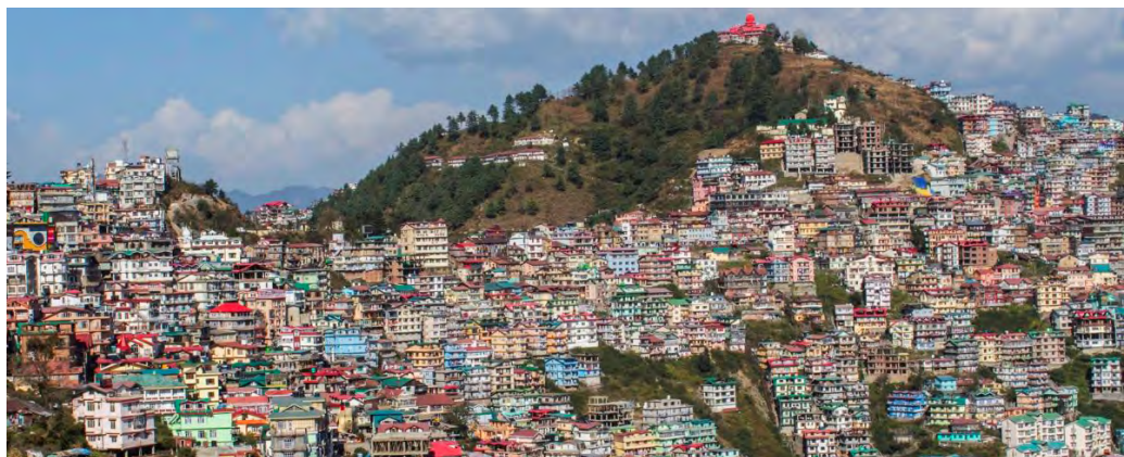
Sanjauli area of Shimla city dotted by recently done construction of RCC Buildings
